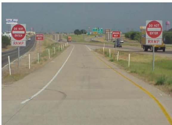
Supplemental placards on ramp
