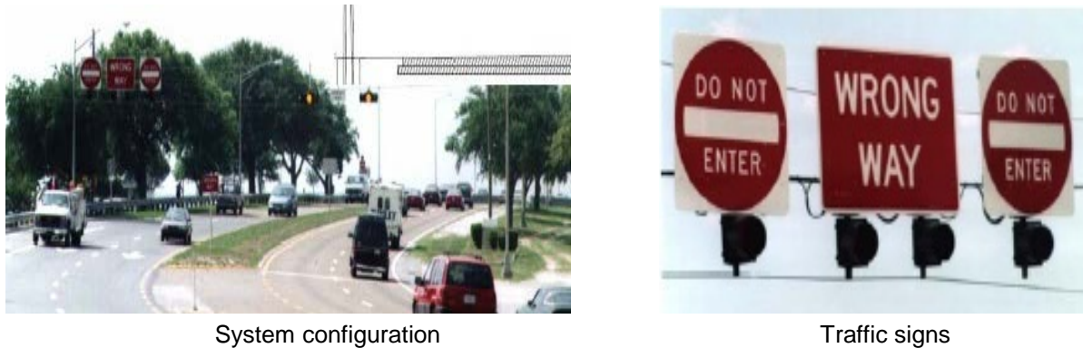
Figure 2.9 Pensacola Bay Bridge wrong-way detection system (Williams 2006).
